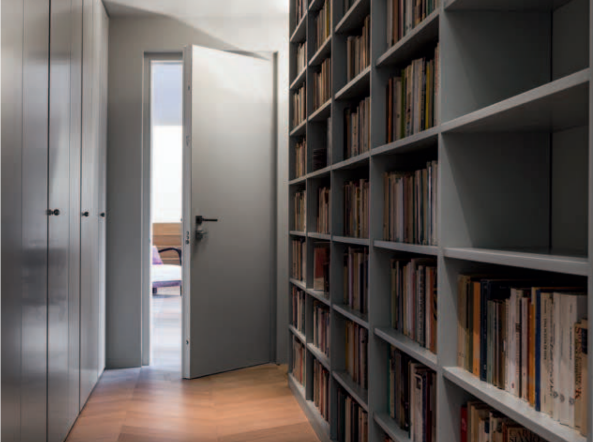
Interior door flush with the internal wall
