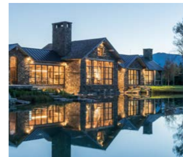
Project: LINN RANCH Architect: JLF Architects
