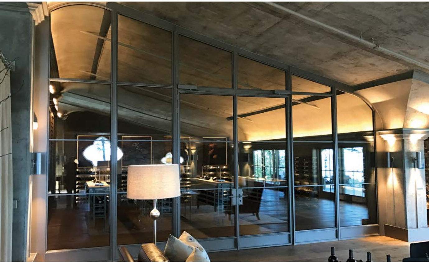
Classy yet literally cool, the Lokoya Winery has large galvanized steel doors by Brombal. The simulated divided lights increase the energy performance, while the narrow sightlines hold large panes of glass. The wine coolers with Brombal doors keep the cold air in and the warm air out.
